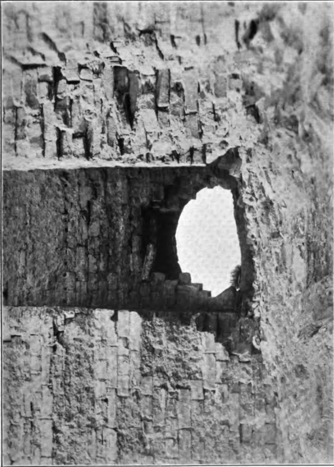
PART OF THE CITY WALL AT SALAHIEH.
